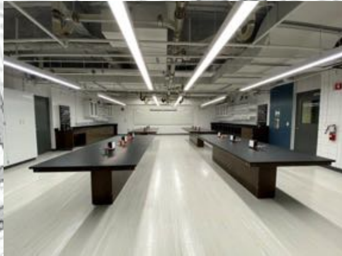
Renovation of Existing Academic Buildings
