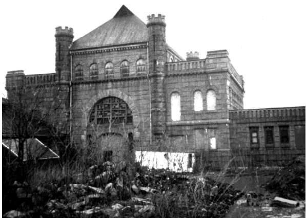
Photo: Calf Pasture Pumping Station, MACRIS Database
