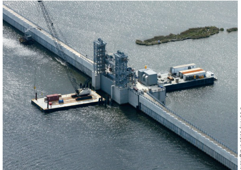
Example of vertical lift gate.
